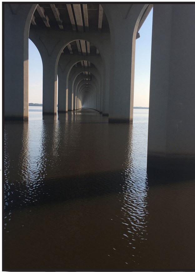
The I-220 bypass loop around Shreveport, LA passes directly over the eastern portion of Cross Lake. Along the bridge piers on the southwestern portion of the bridge, artificial reefs were sank along the even numbered piers from pier 20 through pier 42.
