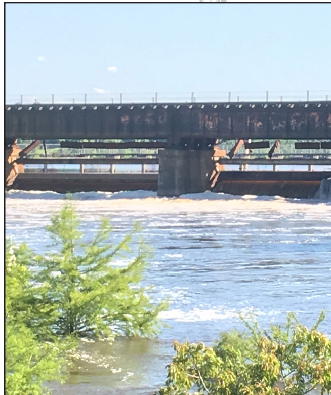
2019 saw Cross Lake reaching over three feet above pool stage. Shown here the spillway with gates open, discharging water into a plunge pool that is nearly the same elevation as the spillway thanks to flooding along the Red River backwaters of Twelve-Mile Bayou and Cross Bayou.
